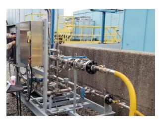
**NOx Reduction and Power Augmentation:** On the Turbine side, Petrotech modified one (1) Set of 10 fuel nozzles/ combustor end caps and to fit new water injection nozzles. Then we installed new WI header and SS water injection manifolds tubing around the combustors where we connected them to the new water nozzles. Also, the manifolds were connected to the main WI header back to the water skid.
